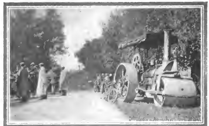
Inspecting a new-laid road en route to Springfield, Mass.
